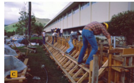
▲ B Design-phase renderings of Sierra Madre Hall. C Students building the concrete Erhart Ag Bridge.
